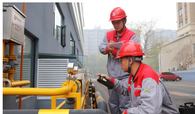
Natural Gas Pipeline Network Maintenance
